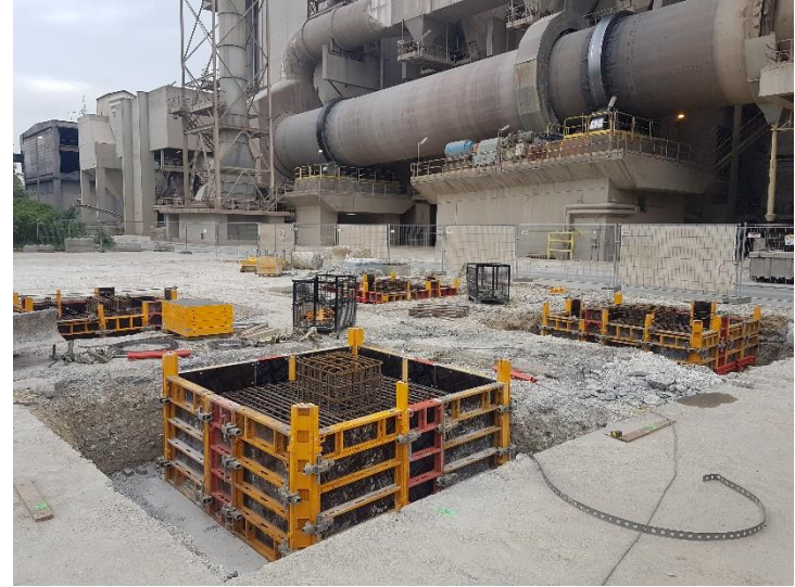
Piles ready for pouring (16 May 2018)
