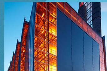
Fortum Oslo Varme AS (Klemetsrud) Waste-to-energy plant
