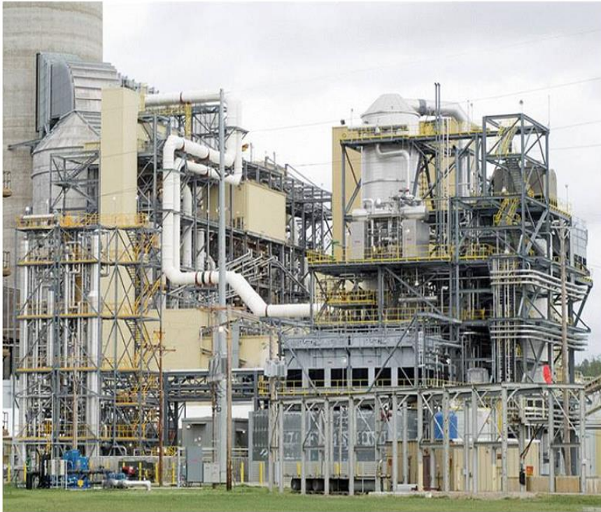
Mountaineer test facility, with a gas flow 25% of CEMCAP standard size
