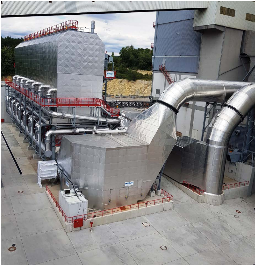
Figure 1: DeCONOx plant in a German cement works
