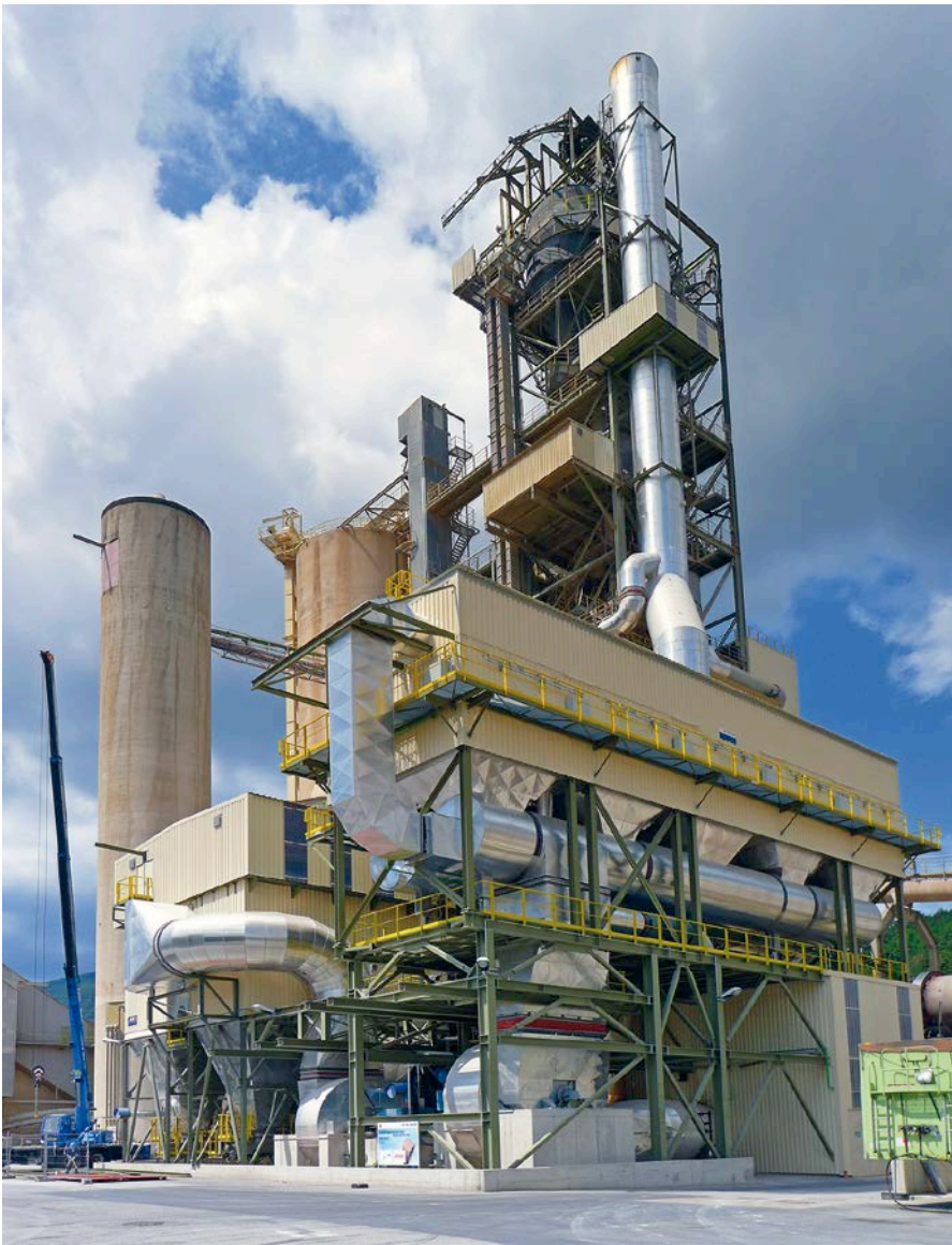
Figure 2: RTO facility in a cement works
