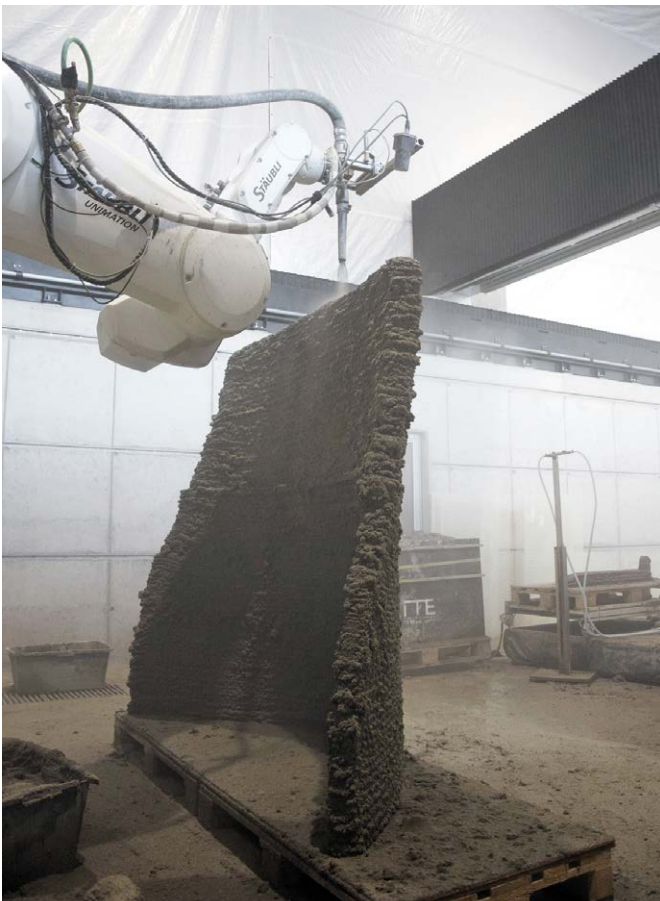
Figure 2: Layer-by-layer construction of a wall with a Shotcrete 3D printer
