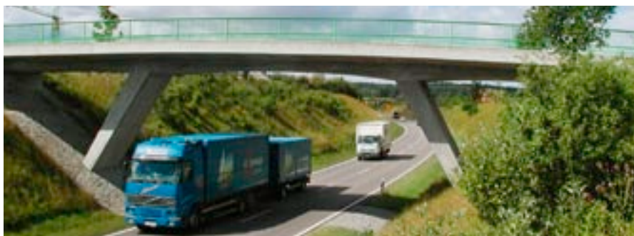
An example of the successful use of CEM II/A-LL 32,5 R: The Merklingen Bridge (Germany), built in 1998.
