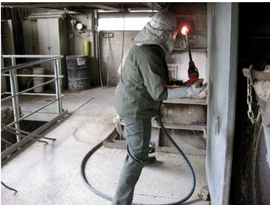
Figure 1: Removing coating with a pneumatic hammer.
