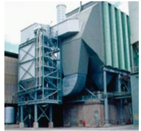
Figure 2: ORC waste heat boiler using cooler exhaust air heat at 275 °C. Source: Jan Theulen: Waste heat power generation at modern cement plants . Verein Deutscher Zementwerke: Process Technology of Cement Manufacturing: 6th International VDZ Congress 2009 , Duesseldorf.
