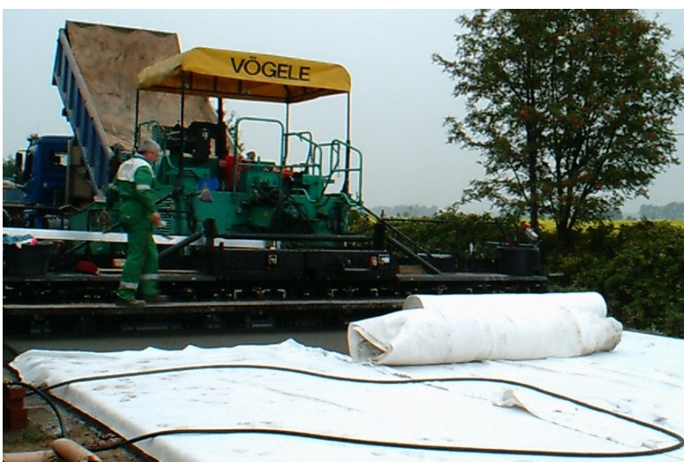
Fig. 1: Spreading of porous concrete with a paver
